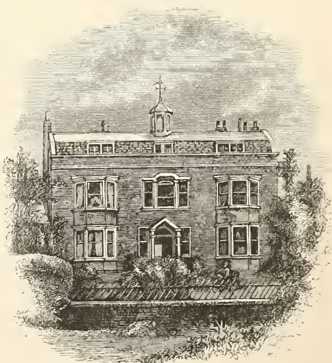
GAD'S HILL PLACE, NEAR ROCHESTER (1860-'70).
